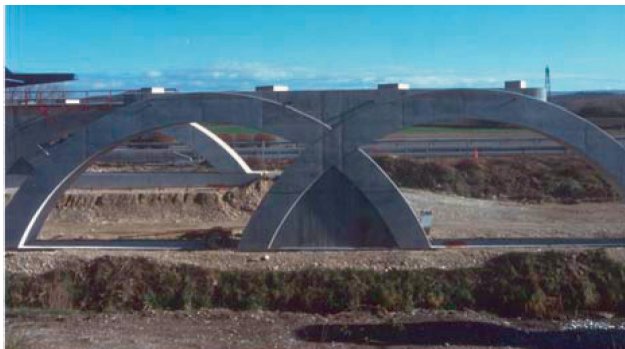
Figure 2. Bridge parapet cast with Formtex®.
